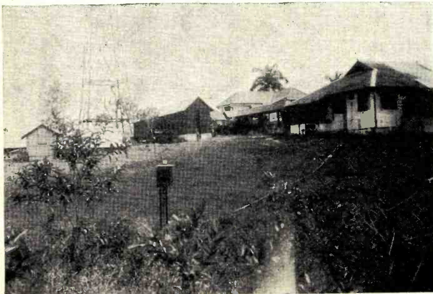
General view of Stations VRR4 (11.595) and VRR5 (12.050), Stony Hill, Jamaica. These stations are used chiefly for relaying sports and other events from SW station ZQI, Kingston. Transmitter building is at right, quarters and storerooms may be seen in center of photo.
